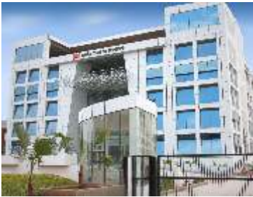
Office at Chandigarh
